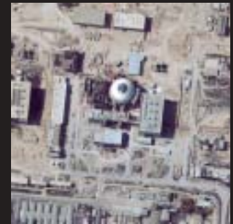
Bushehr nuclear facility - Iran
